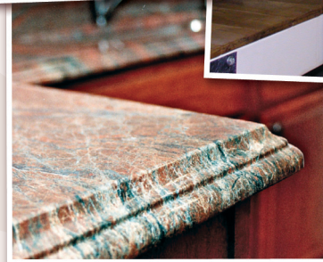
Two layer edge profile: Ogee with 3/8" Bullnose
